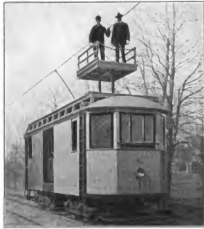
Fig. 227. Reparaturwagen der Old Colony Street Railway Co.
